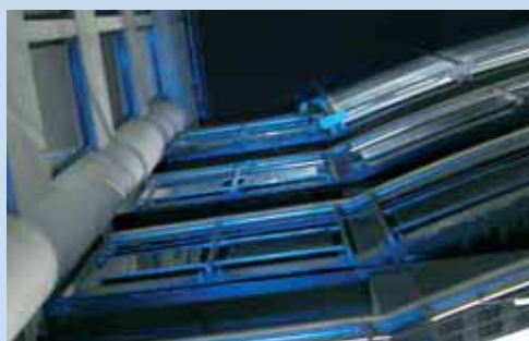
B O U L O G N E - France Car park - 4540
