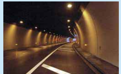
O R E L L E S - France A 43 - Sorderettes Tunnel - 1821
