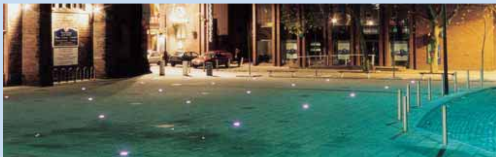
W A L S A L L Walsall Bus Station - St-Paul's Church Square - AHMM Architect - 2852
