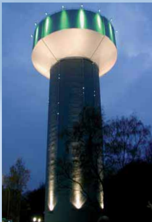
C A N T E L E U - France Water tank - LIGHTEC - 1826
