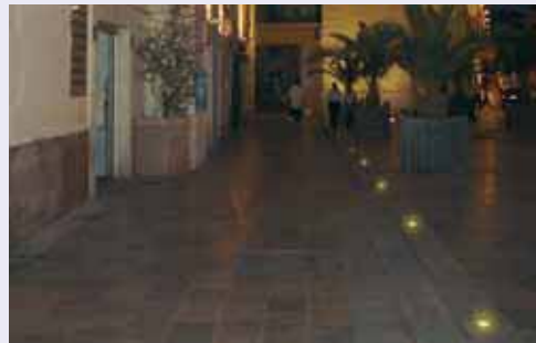
NÎMES - France The access to the tower is marked with recessed marker-lighting with dynamic colours programmed on a pre-defined scenario - 1830
